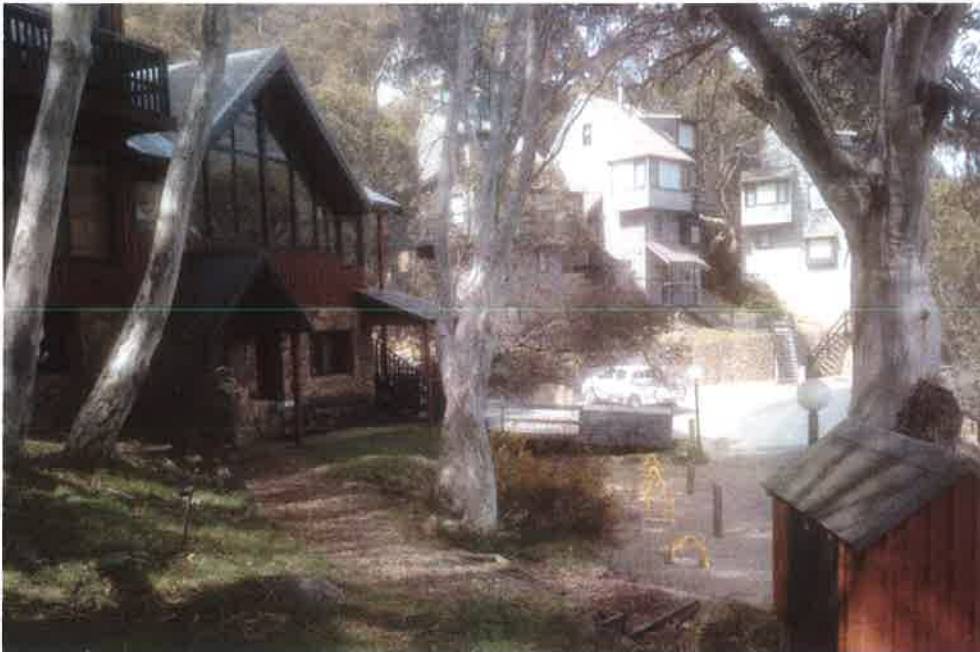
Photo 2 – View of the front of lodge from the east
